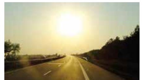
The effects of weather: stresses caused by thermal fluctuations due to exposure to direct sunlight during the days and drastic cooling down in shady areas or at nighttime.
