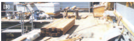
Illustrations: [1] metalwork; [2] roofing felt nail; [3] flat roof used for storage
