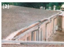
Illustrations: [1], [2] damage by cold contraction
