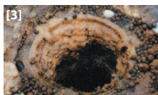
Illustrations: [1] material failure below gravel; [2] low-quality mortar; [3] sintering inside roof drains
