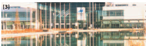
Illustrations: [1] air-conditioning unit on a flat roof; [2] embrittlement of roof sheets; [3] sealed pond on Munich's trade fair premises
