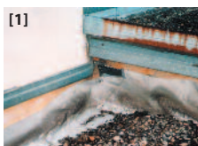
Illustrations: [1], [2] damage by cold contraction
