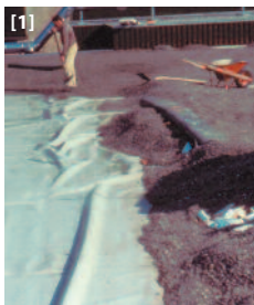
Illustrations: [1] material failure below gravel; [2] low-quality mortar; [3] sintering inside roof drains
